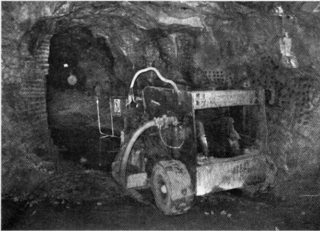
Machinery in the Camborne School of Mines (former Holman Brothers) Test Mine. Photo: Roger Starling
